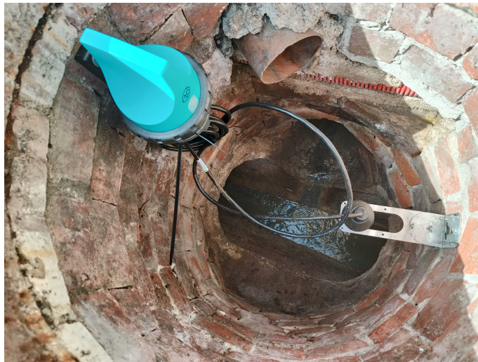
Figure 2.1: Sensor deployment in a wastewater network maintenance hole for flow monitoring purposes. Source: Cicle de l'aigua del Ter.
